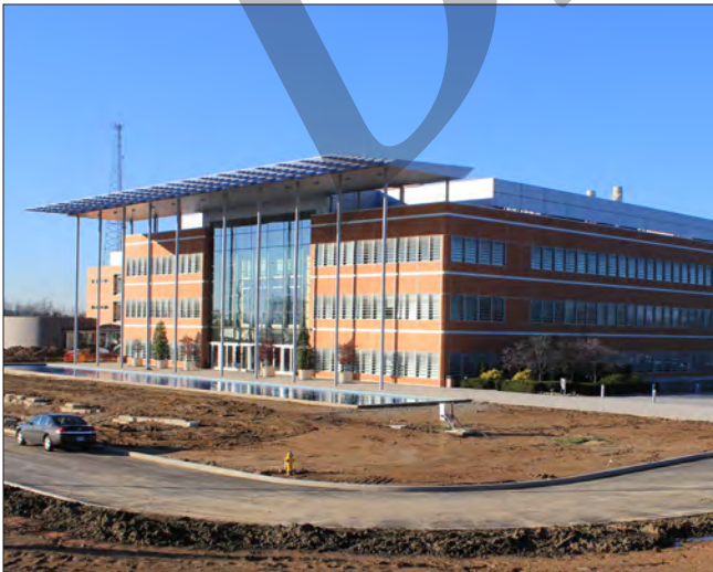
DONALD DANFORTH PLANT SCIENCE CENTER
