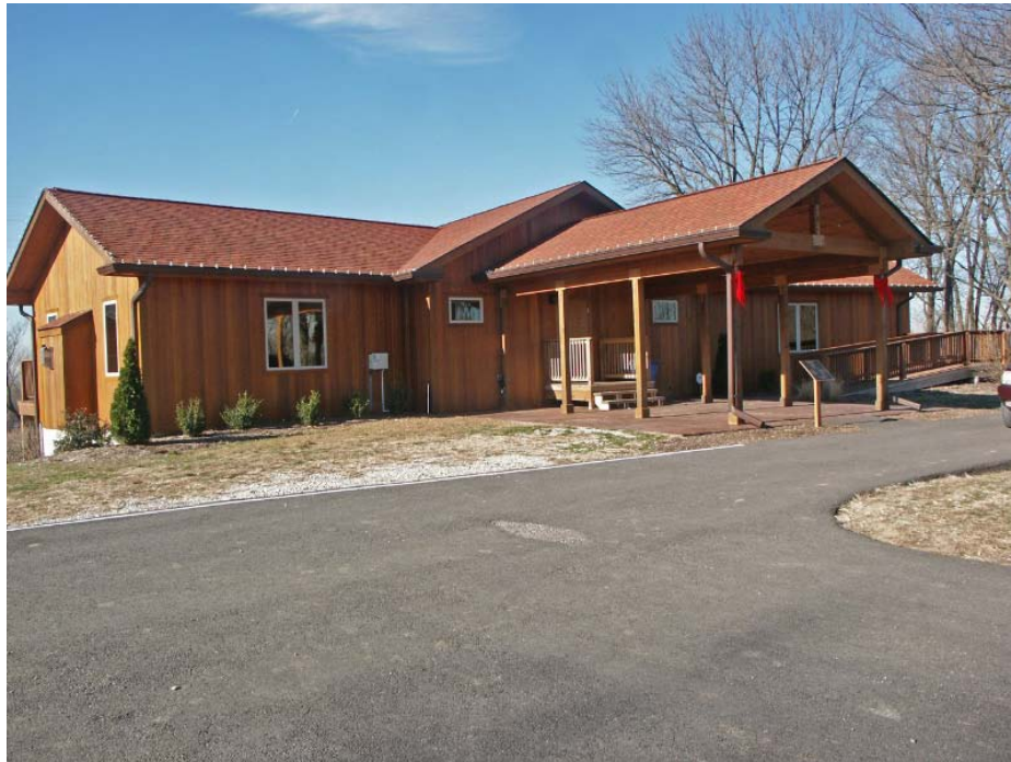
Construction Completed May 2009 of the Nature Lodge at Sunset Park.
