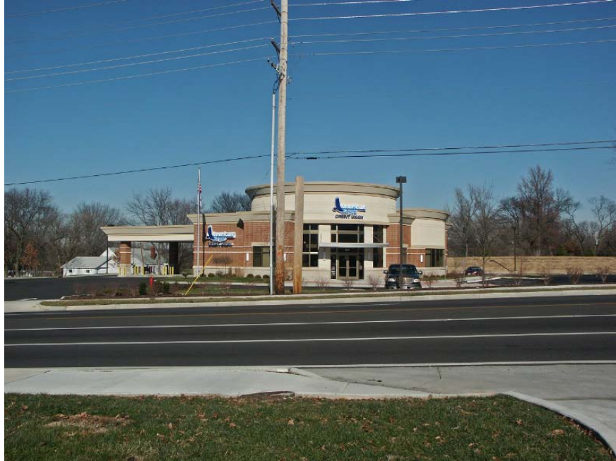
Construction was completed November 2009 for the Eagle Credit Union, 1150 North Highway 67.
