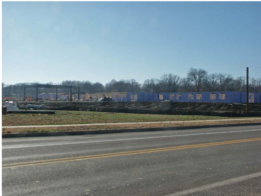
Construction began August 2009 for the Garden Plaza Care Center, 2300 Parker Road.
