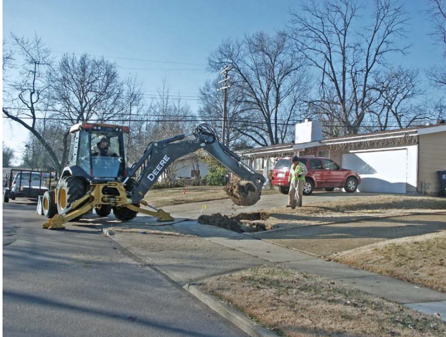
Excavation of a Residential Sanitary Sewer Lateral by City Employees.
