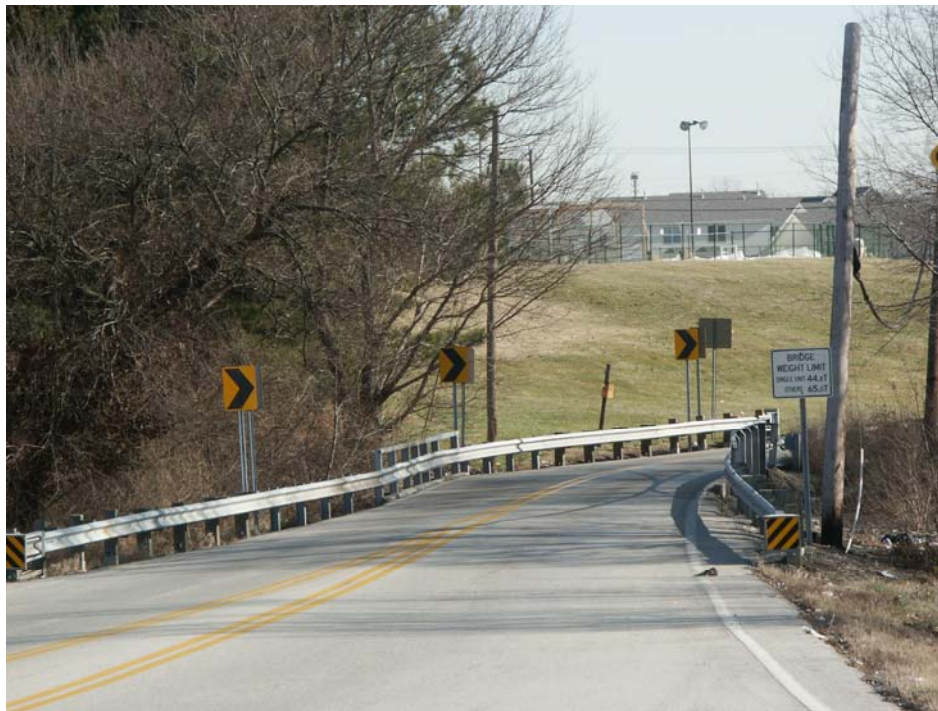
Existing Greenway Chase Drive Bridge Scheduled for Replacement in 2011.
